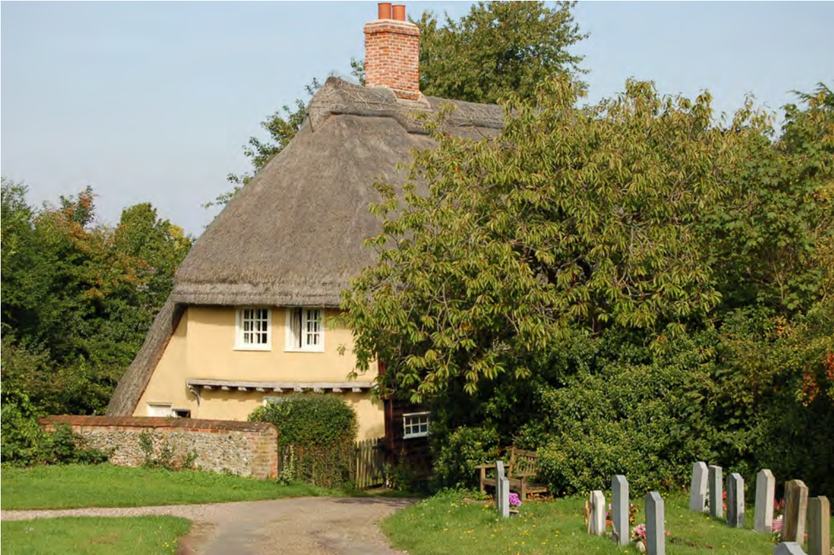
Picture 1.14 Beam Ends; a quintessential English cottage, attractively colour washed, thatched and with small neat horizontal sliding sashes. It sits on the rising path to the church
