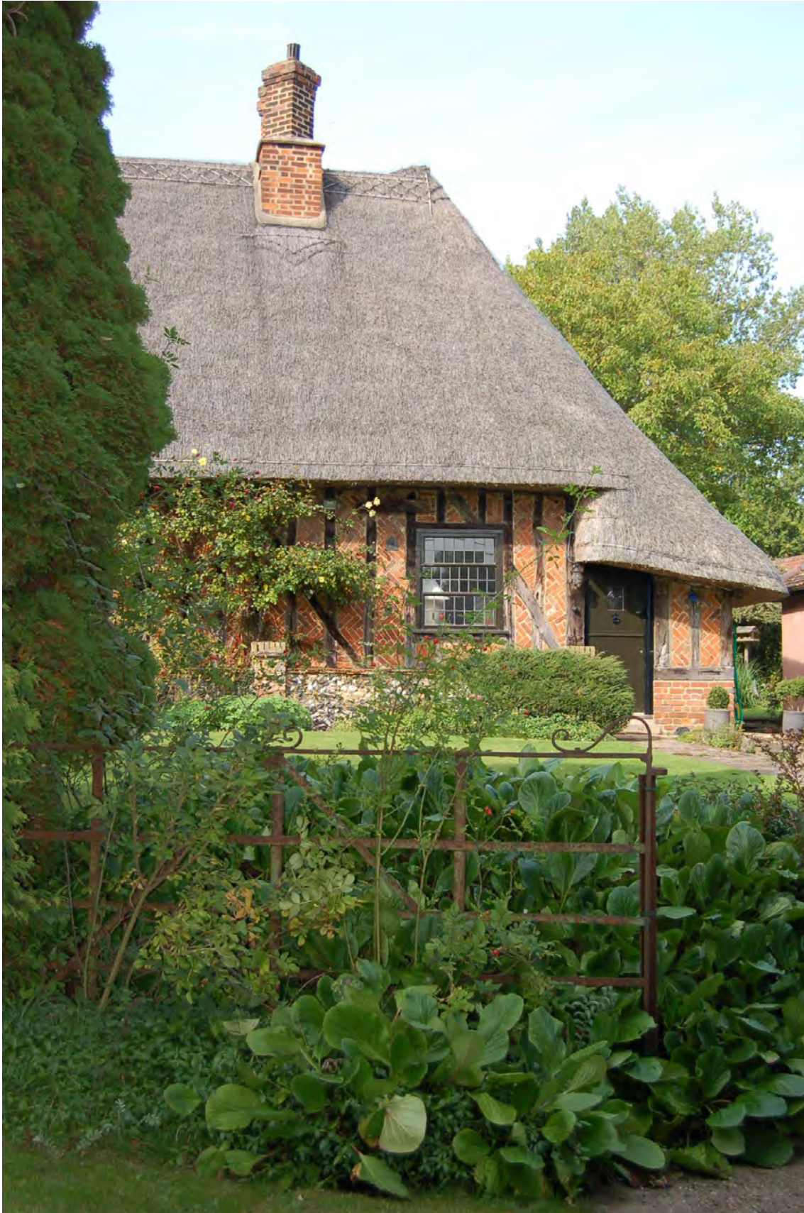
Picture 1.17 A low thatched roof, contrasting brick nogging and decorative chimney treatments presents a most pleasing aspect
