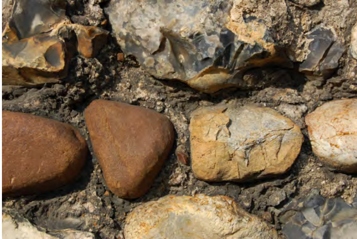
Picture 1.8 Traditional Essex flint panelling on the wall linking Kings Cottage and Walnut Cottage
