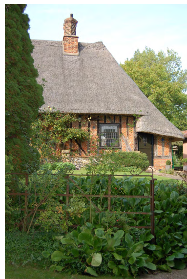
Picture 1.7 Brick nogging employed to dramatic effect as an infill on Dormer Thatch
