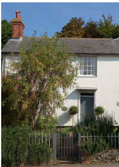
Picture 1.6 Slate, white-washed plaster and simple iron railings on a half height flint wall in Linton Road
