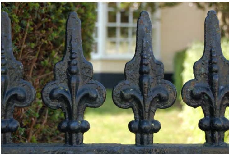
Picture 1.9 Listed railings to the front of Yew Farmhouse
