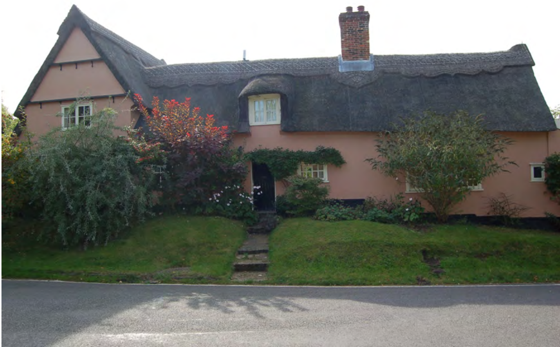
Picture 1.16 Hillcrest Cottage completes the varied progression of properties up Bartlow Road
